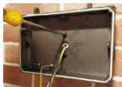
2. Mount rear portion of mounting box to junction box.
