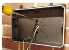
2. Mount rear portion of mounting box to junction box.
