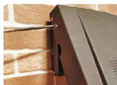
5. Adjust desired angle and tighten the set screw for angle adjustment to lock.
