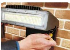
4. Place front of fixture against rear portion of mounting box and tighten previously removed screws to secure.
