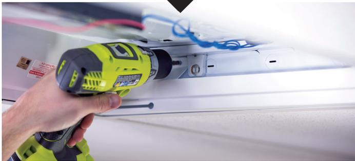
3. **Optional:** Install side plates (x2). This is dependent on whether or not there are gaps between the fixture and the existing ceiling grid.
