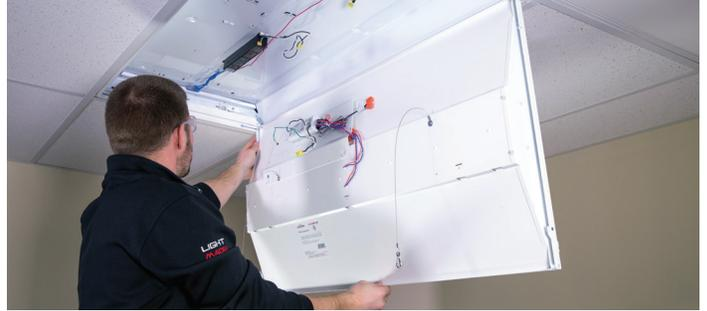
5. Hook safety cables into existing lances/holes of the fixture.
