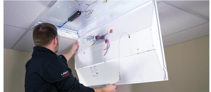
**5. Hook safety cables into existing lances/holes of the fixture.**
