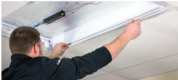
**4. Insert the doorframe of the retrofit into the keyholes of the support brackets and slide the unit into place.**
