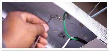
**5.** Make electrical connections for input power (via the included Power Quick Disconnect) and fixture ground. 0-10V connections optional.
