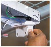
**3.** Break apart the 1-piece mounting bracket kit into 2 individual pieces. Install the brackets to each end of the fixture by bending them over the fixture to fit the exact width and fastening them to the fixture with the provided tek screws.
