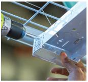
**4.** Fasten the safety cables (x2) from the retrofit pan(s) to the fixture housing using existing lances/holes of the fixture.
