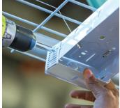
**4.** Fasten the safety cables (x2) from the retrofit pan(s) to the fixture housing using existing lances/holes of the fixture.
