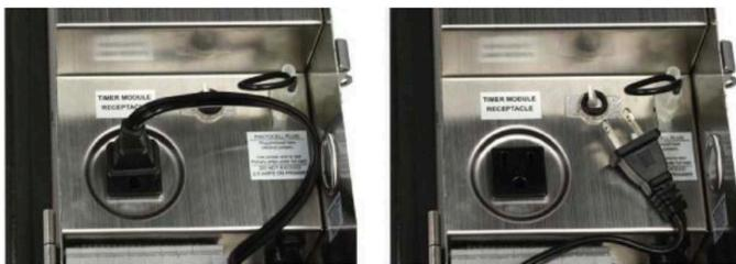
1. Disconnect the power source from the transformer before installing the timer
