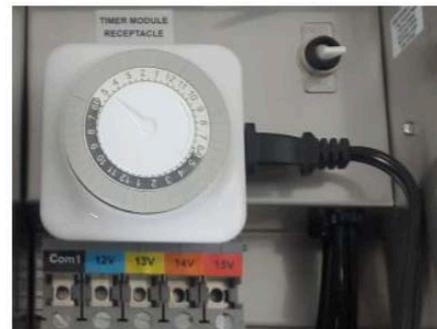
4. Insert the timer into the outlet on the transformer as shown on the above picture
