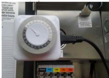
3. Insert that plug into the side of the timer as shown on the above
