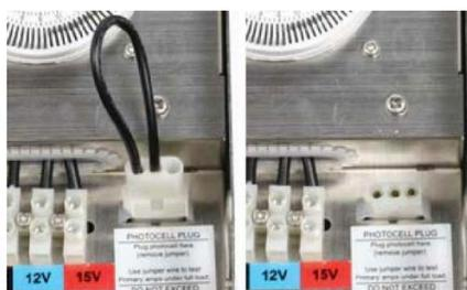
Unplug the jumper connection from the transformer
